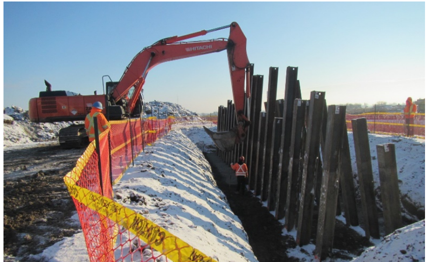
Highway 427 Bridge Construction (January 2019)
