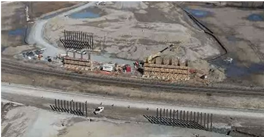
Photo of construction from March 2019 drone footage at CP Railway/McGillivray Road
