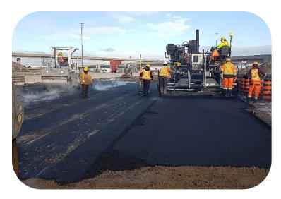
**Paving Machine:** A paving machine lays asphalt and concrete on the road surface. The machine will move at a constant pace to ensure that the surface is smooth.
