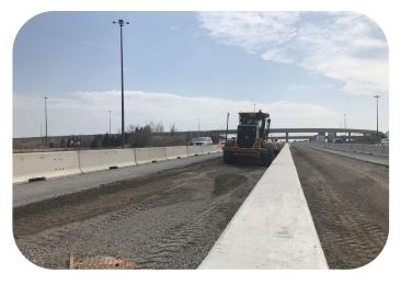
**Grader:** This machine will flatten the road with a long blade to create an even surface for a paving machine to lay asphalt onto. Pictured on the left, this grader is preparing the median for paving on Highway 427.
