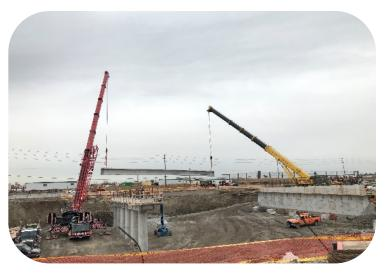
**Cranes:** Cranes will lift girders which are steel beams onto the bridge piers (columns). Girders will support the bridge deck which is the surface of the bridge. Pictured on the left, two cranes are lifting girders onto the new bridge structure at Langstaff Road.
