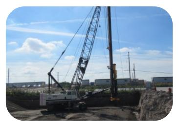
**Pile Driver:** Piles (poles) are driven into the ground to support the weight of structures. Pile drivers are cranes that hammer the poles into the ground. Pictured on the left, piles are being hammered into the ground at the new Langstaff Road structure.
