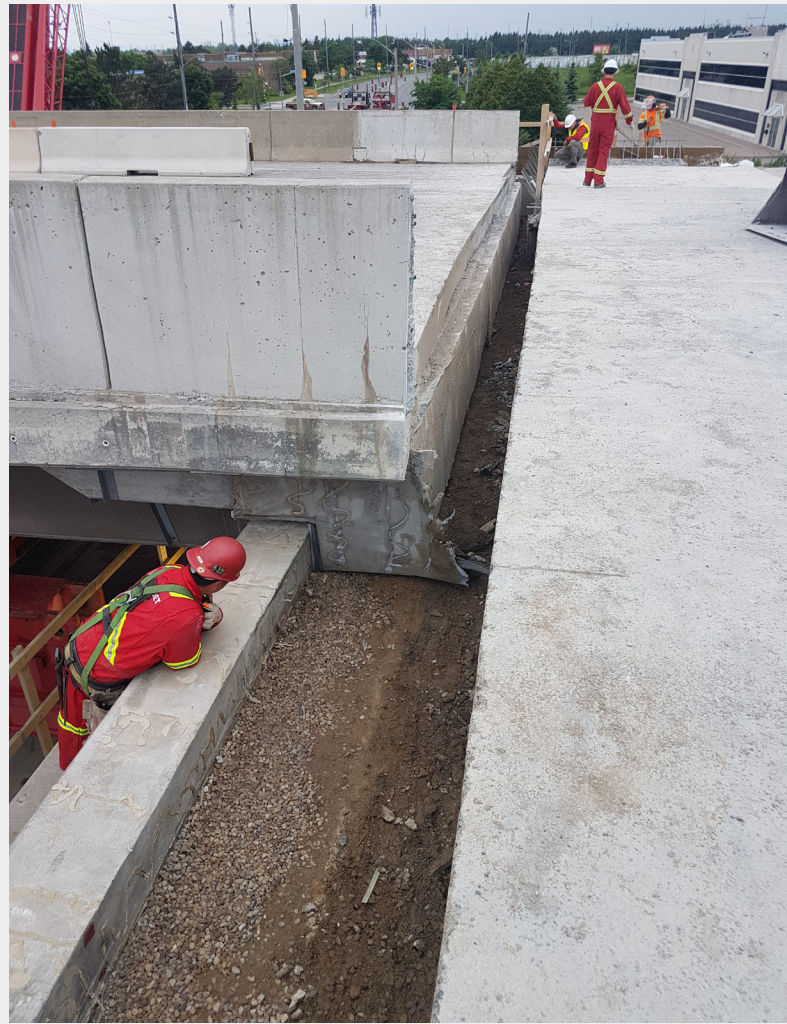
View of Albion Road bridge move near completion.
