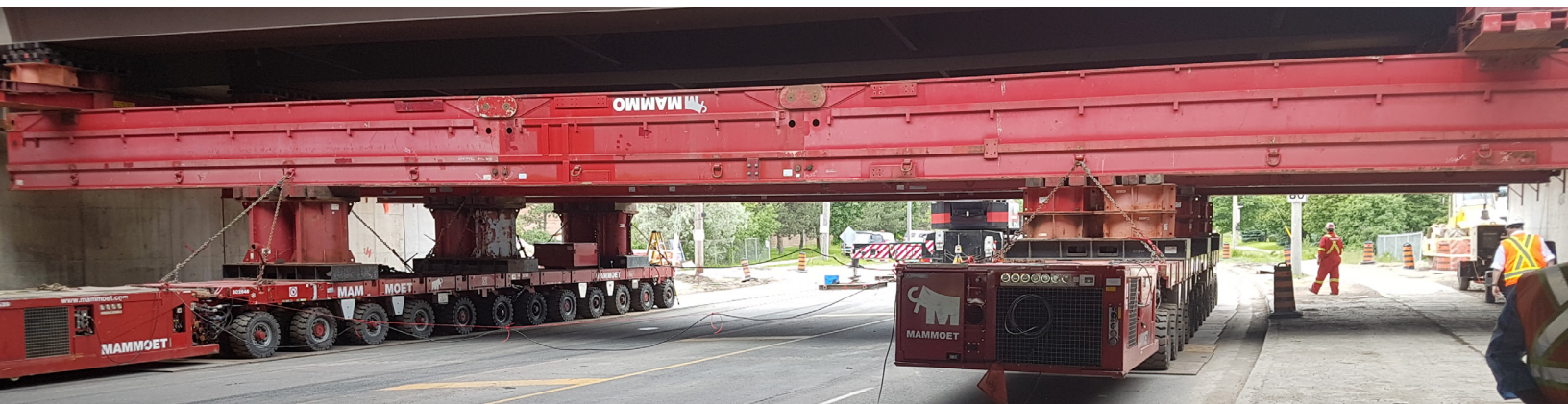
View from Hwy 427 of Self-Propelled Modular Transporter machine set up below Albion Bridge on Saturday June 16 prepared for the bridge move.
