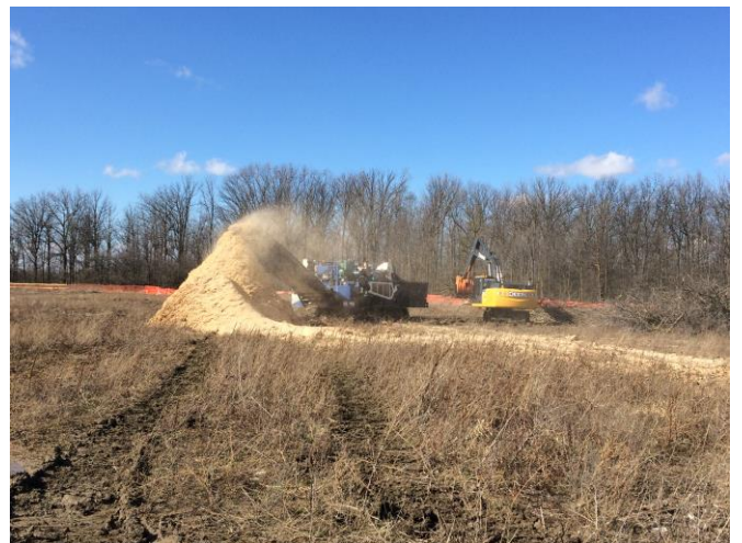
February 26, 2018. Clearing operation north of Langstaff Rd. Grinding of tree material. Some of the wood chips will be spread on the ground to reduce erosion.
