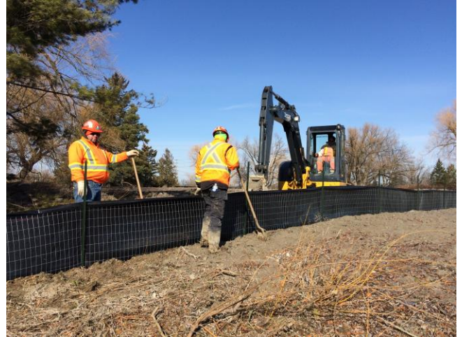
February 27, 2018. Installation of Environmental Controls, south of Rutherford Rd. Steel-mesh fence controls sediment flow from preloading sites.
