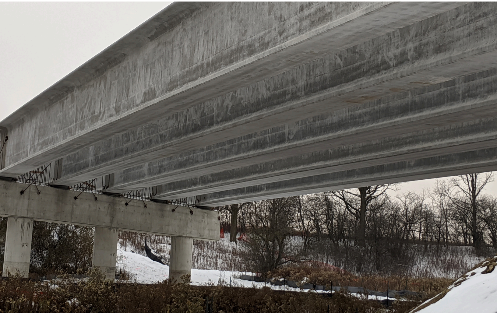
Girders installed over West Robinson Creek.
