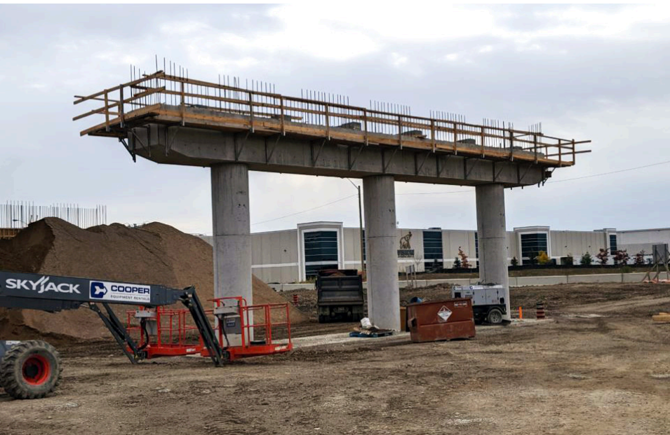
Pier construction for the future alignment of Zenway Boulevard.
