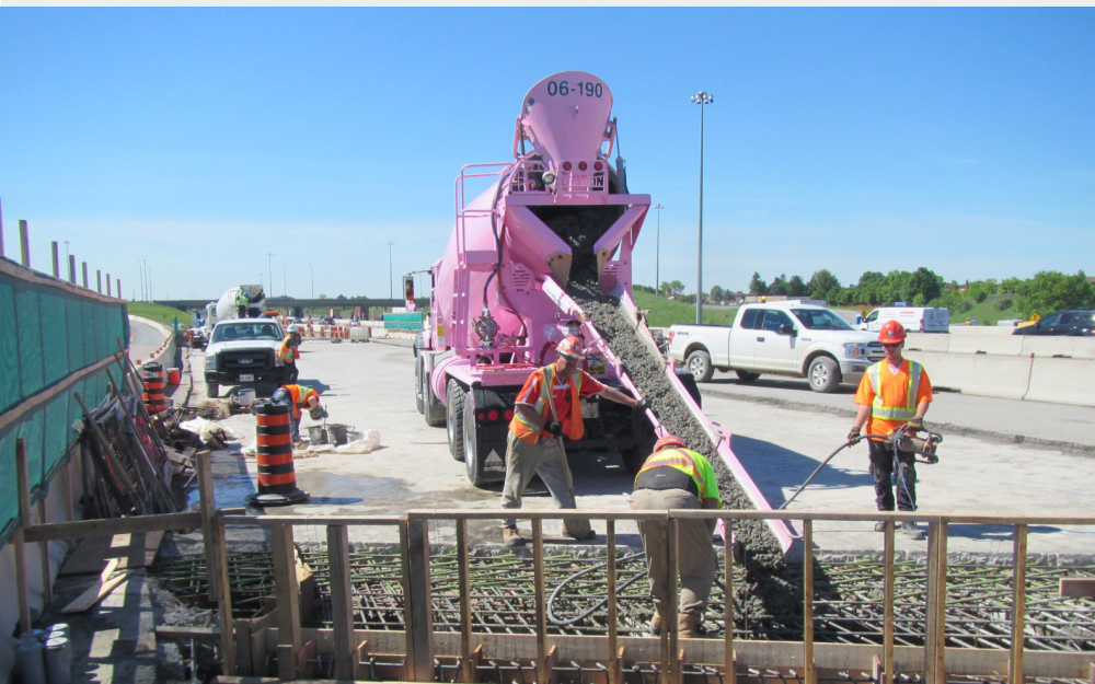
Workers pouring concrete in the northbound lanes of Highway 427.
