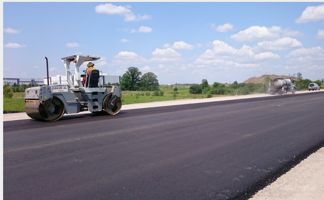
Paving work north of Zenway Boulevard.
