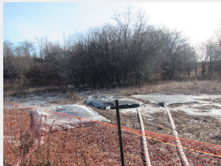
Dewatering station with sediment bags near Rainbow Creek.
