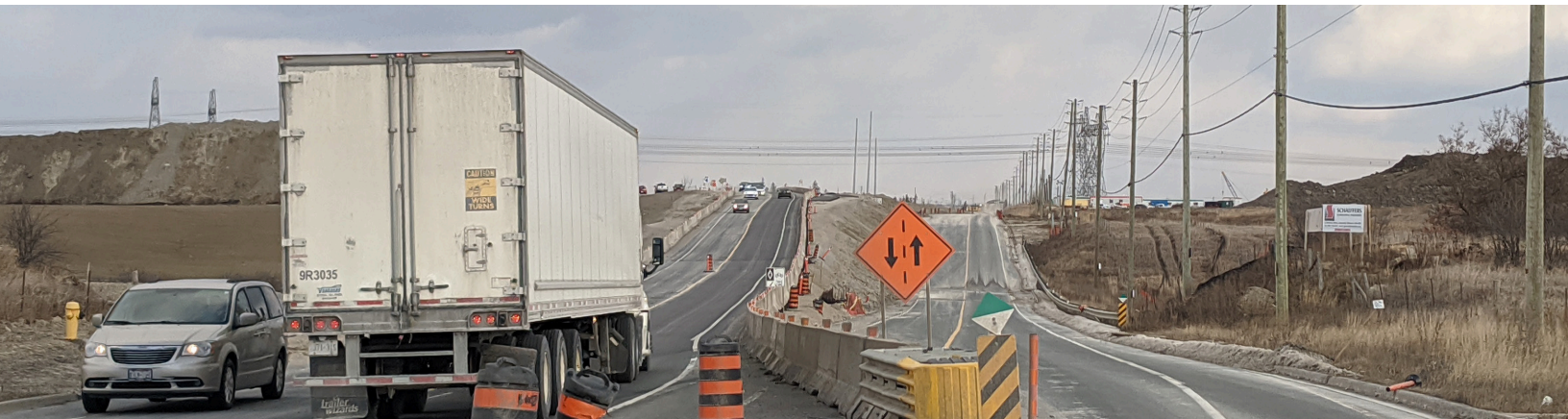
Vehicles driving on the new alignment of Langstaff Road. The old alignment of the road can be seen in the right half of the photo. Langstaff Road was shifted on November 29, 2019.
