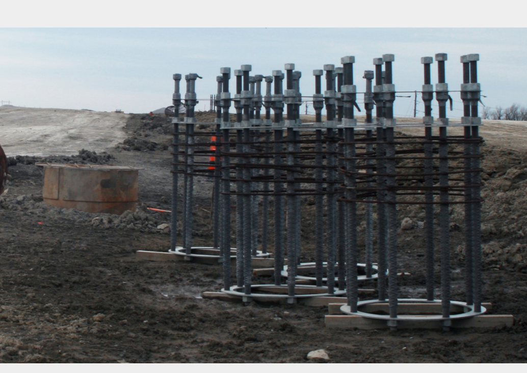
Rebar for the base of high-mast light pole.
