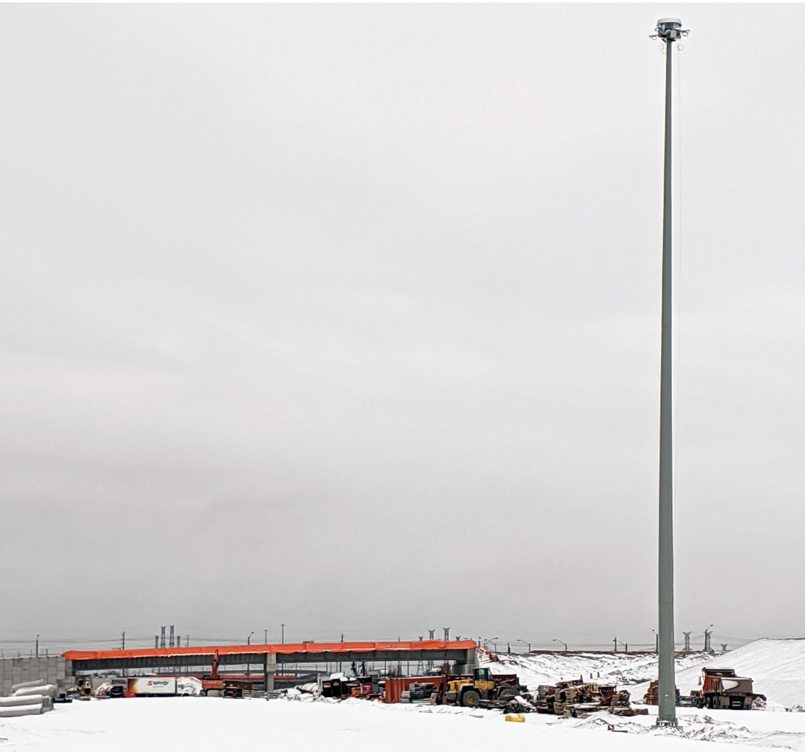
Newly installed high-mast light pole near Rainbow Creek.
