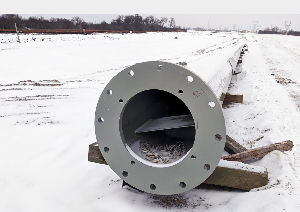
High-mast light pole ready for installation on the Highway 427 Expansion between Rutherford Road and McGillivray Road.
