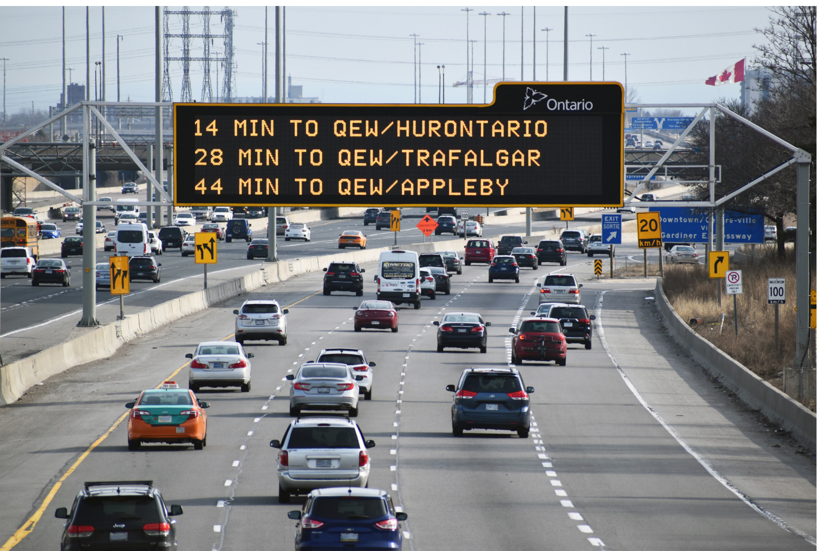
A variable message sign above the southbound collector lanes of Highway 427 near Burnhamthorpe Road in Toronto, showing travel times.
